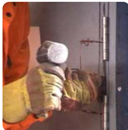
Attacking the door with a chisel and mallet to remove the skin.
